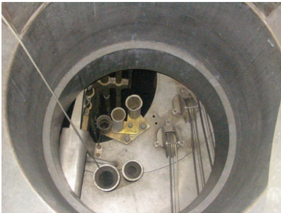
Figure 3. Lowering the 612-10 FHZ probe into the HC1 through the channel 43/4
