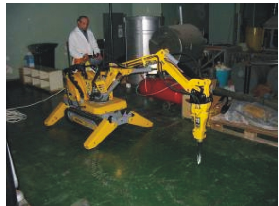
Figure 7. Remote radio-controlled demolition equipment
