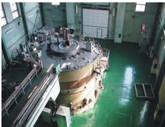
Figure 1. VVR-S research reactor in Magurele
