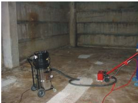
Figure 9. Scarifying equipment for the decontamination of floors and walls by compressed air supply
