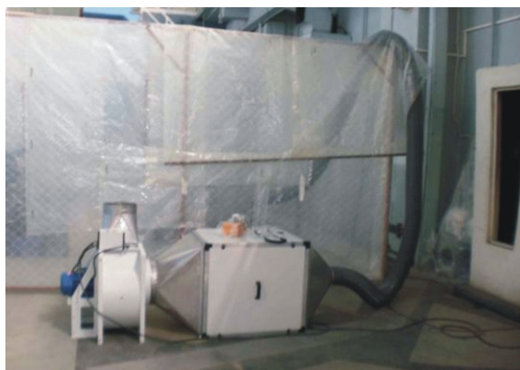
Figure 3. Temporary tent and ventilation
