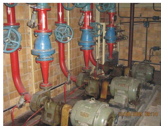
Figure 6. Cooling loop prior to the dismantling
