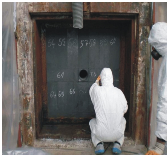
Figure 9. Graphite from the removal of the thermal column
