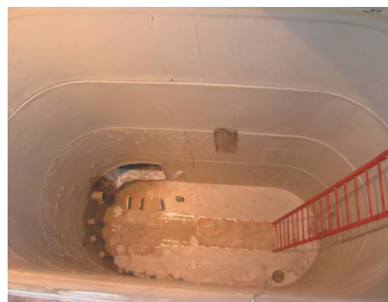
Figure 5. Reactor pool after the dismantling
