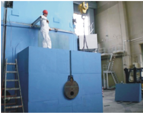
Figure 8. Thermal column prior to the dismantling
