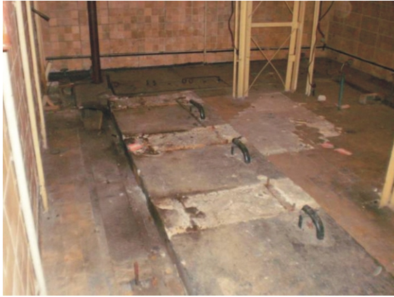
Figure 7. Cooling loop after the dismantling
