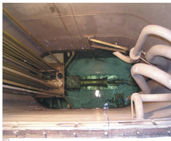
Figure 4. Reactor pool prior to the dismantling
