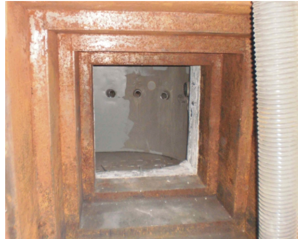
Figure 10. Thermal column after the dismantling
