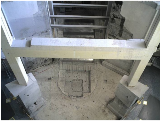
Figure 2. View into the empty reactor hall of SAPHIR after the removal of the reactor
