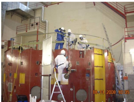
Figure 3. View onto the remaining lower part of the shielding of DIORIT reactor
